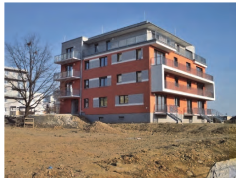
Figure 7 The studied multi-family residential building. Completed building
