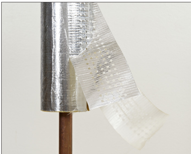
Figure 7. The longitudinal joints should be sealed with perforated aluminium tape to ensure that the joint is closed
